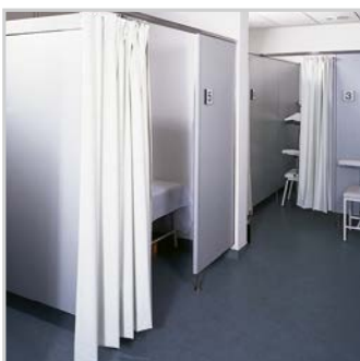
Treatment rooms with either a door or with curtains, vestibule partitions and other rooms solutions.
